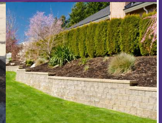
STABILIZATION FOR RET. WALL FOOTING
