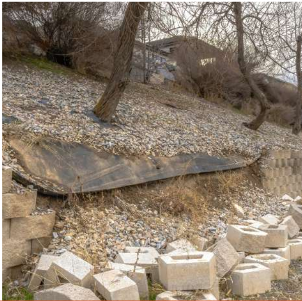
WITH NO GEOGRID INSTALLED
