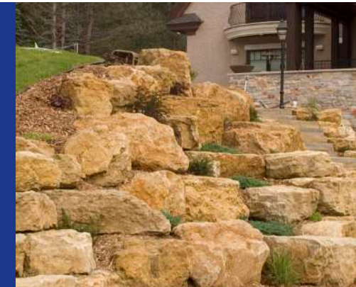
BOULDER RETAINING WALLS
