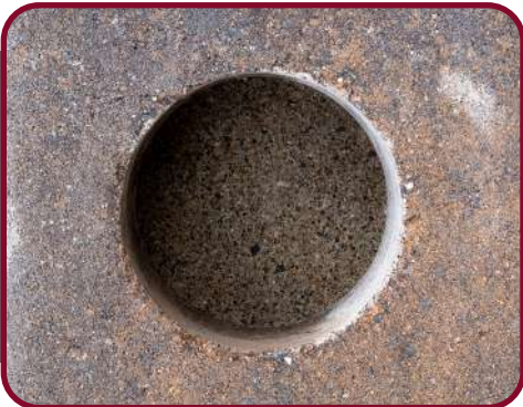
High PSI Concrete
