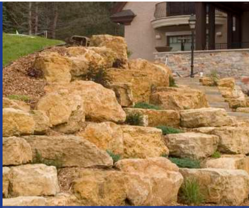
BOULDER RETAINING WALLS
