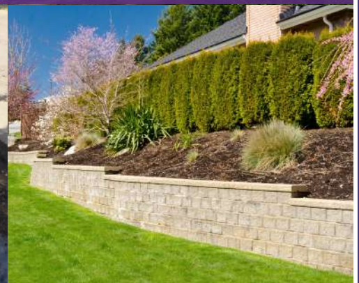
STABILIZATION FOR RET. WALL FOOTING
